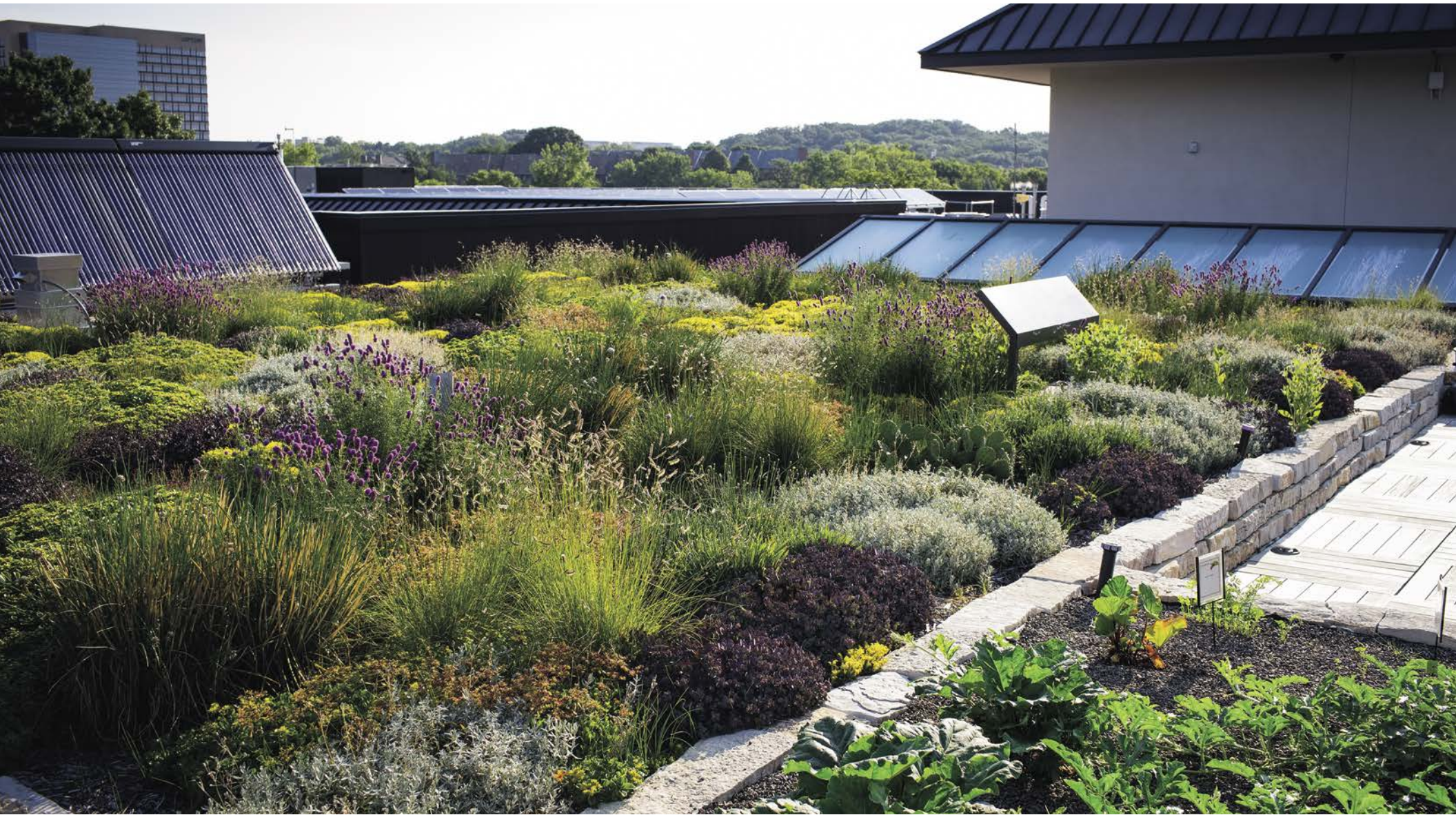
TOP: A green roof and garden make up a portion of the rooftop at the Philanthropies headquarters. This helps insulate the structure below and reduces stormwater runoff, which can contribute to erosion and poor water quality.
